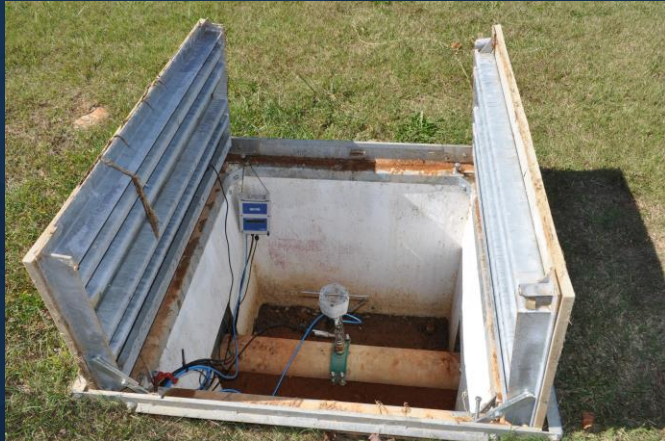
FRP Vault w/ Lockable Hatch
