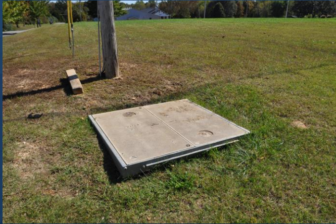
FRP Vault w/ Lockable Hatch
