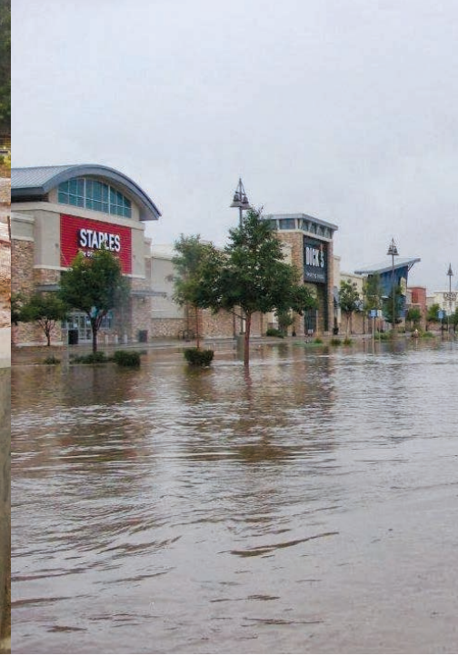
Widespread flooding left residential communities and commercial properties completely inaccessible.
